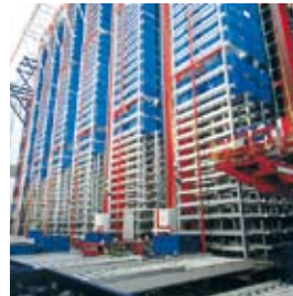
The modern high-bay warehouse ensures efficient logistics
