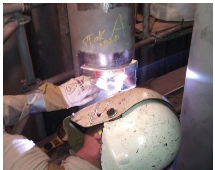
Trained specialist installing a tubeskin thermometer
